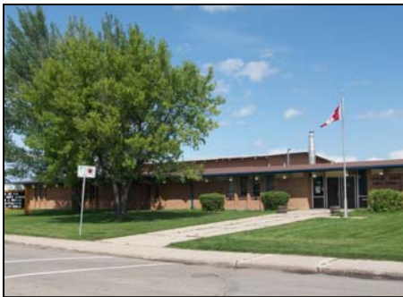
Crosswalk at Caroline Robbins Public School
