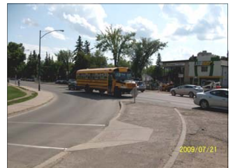
Graded curb cut
