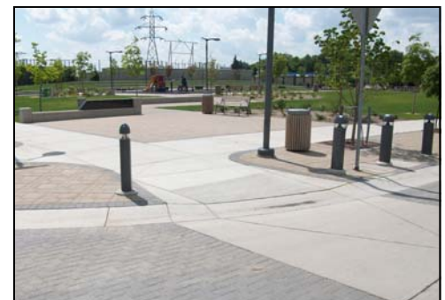
Graded curb cut
