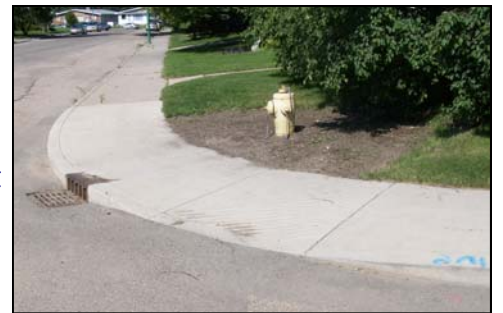
Graded curb cut
