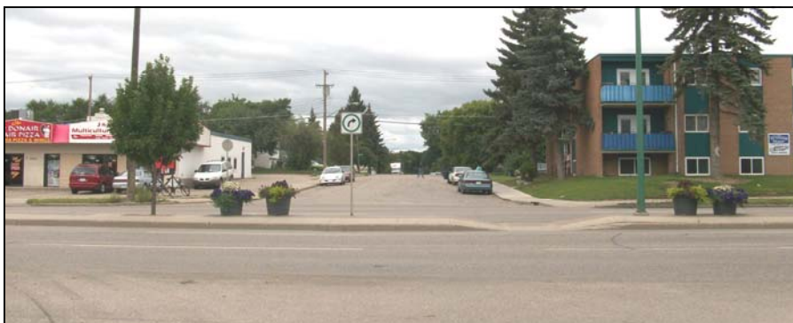
The curb cut in the Pedestrian Refuge enables cyclists to cross the street
