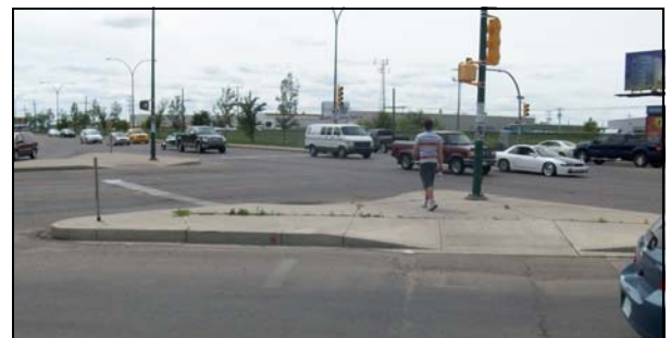
Graded curb cut
