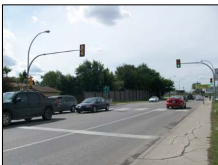
Pedestrian crosswalk in high traffic
