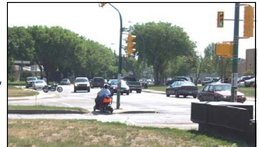
A curb cut in the median enables crossing for individuals with reduced mobility
