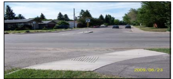
Graded curb cut
