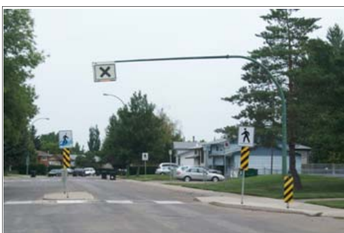
Pedestrian crossing with overhead illuminated sign and traffic calming features
