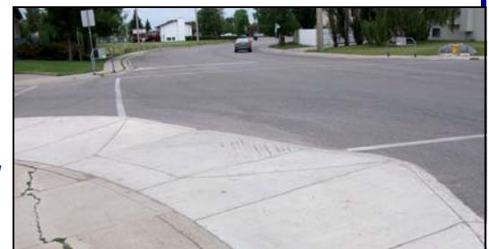
Graded curb cut
