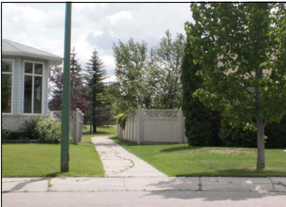
Pedestrian access way
