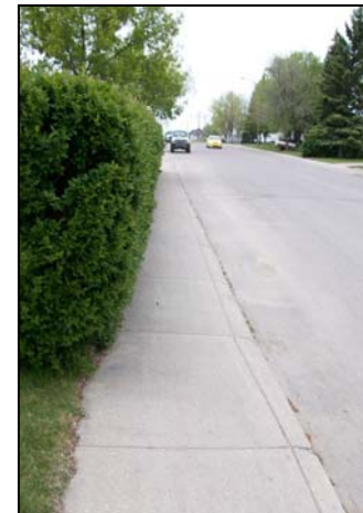
Bush obstructs sidewalk
