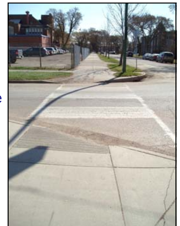
Curb cuts at the crosswalk
