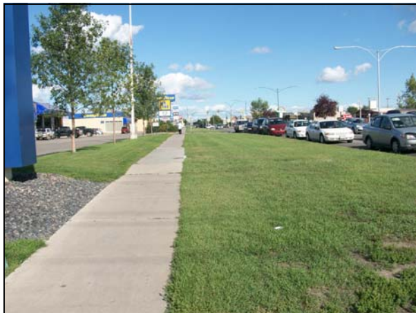
Buffer strip along sidewalk
