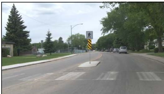
Well marked pedestrian crossing
