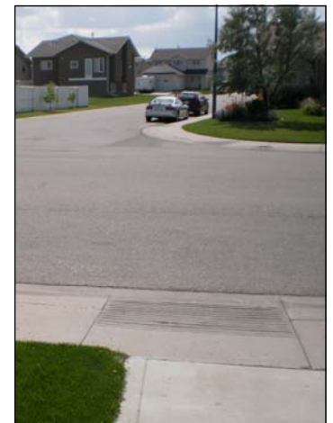
Graded curb cut
